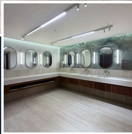
Dekton vanity tops and superloo troughs with Roma Walnut Fascia's. Bespoke mirrors with trims
